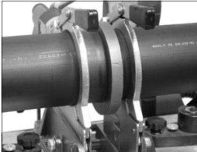
Heating with the heating plate
