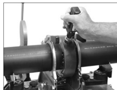
Planing the pipe ends
